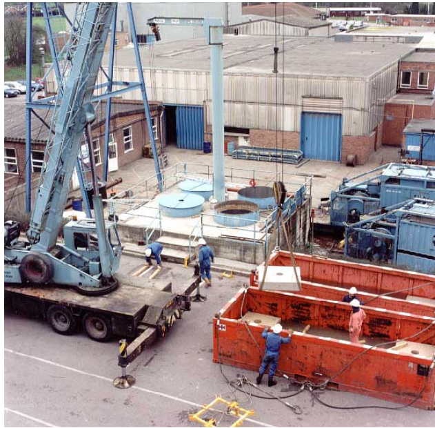
Figure 1. General view of site during rock installation, showing the transit tanks.
