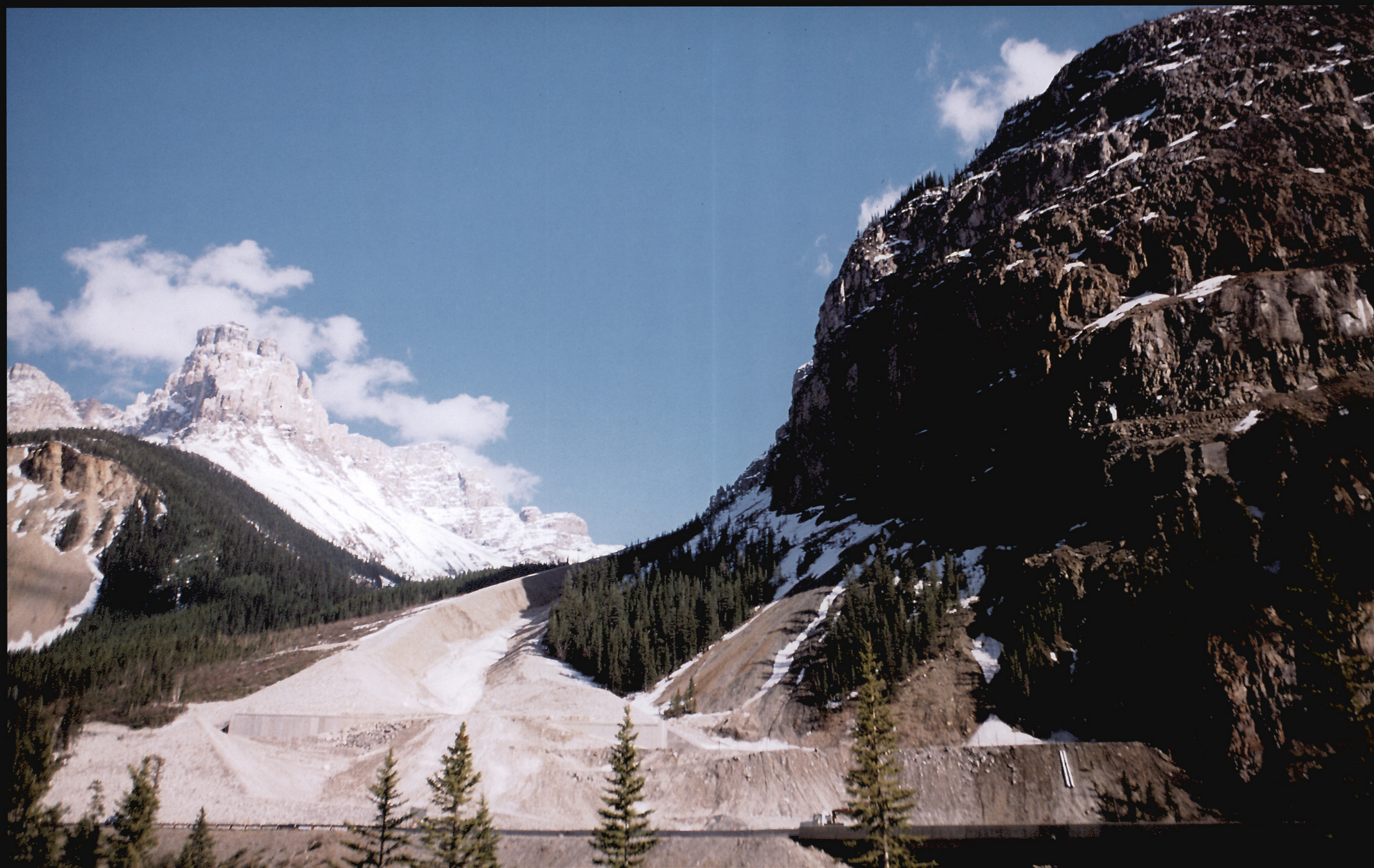
Frontispiece 34.0 Industrial and metallic minerals. Earth works for avalanche diversion around the CPR main line and the Trans Canada Highway on the shoulder of Mount Stephen (right), Yoho National Park near Field, British Columbia. Mount Cathedral in the distance. The rip rap is made up of gangue material derived from (now abandoned) portals located in the cliffs above the scree line on Mount Stephen. The Monarch Mine is a MVT lead-zinc-silver orebody in the dolomites of the Middle Cambrian Cathedral Formation. Closed in 1952, it was one of several mines permitted to operate in National Parks in the early years. Photograph by W.N. Hamilton.
