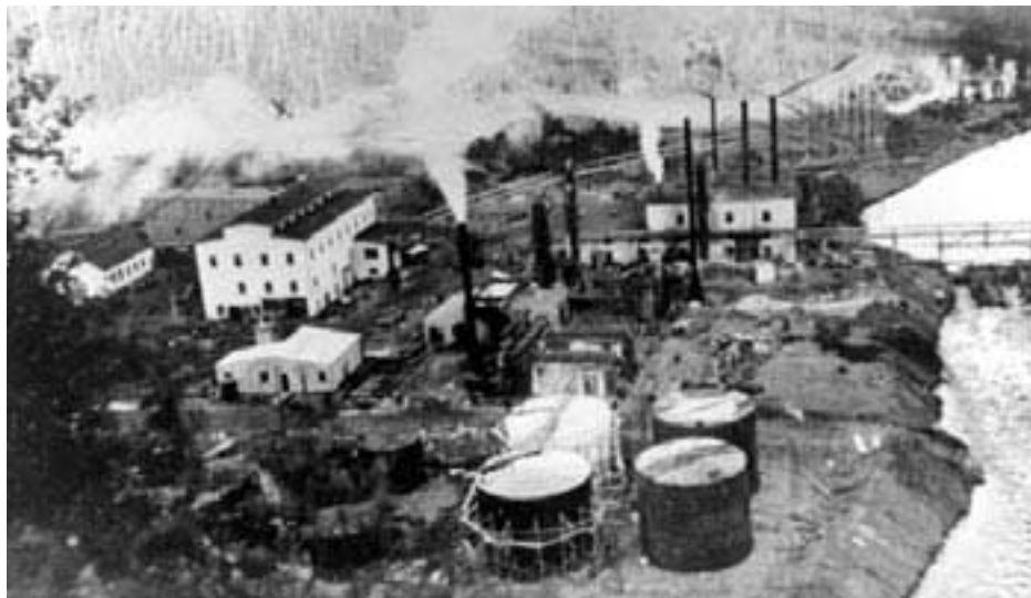
Aerial view of Abasand Oils' plant taken June 15, 1945; the date it is reported to have been destroyed by fire. Apparent cloud in upper right left background marked "X" on photograph may be smoke from the initial blaze. The fire commenced at the loading ramp adjoining the large building to the left of centre which housed the separation unit. This plant, financed by the Dominion Government as a wartime measure, commenced operation in September, 1944 but was incapable of attaining its projected output of 600 tons per day of bitumen. In 1948 the Alberta Government also financed the building of a 500 ton per day plant at Bitumount utilizing K. A. Clark's hot water process. It too was short-lived. Credit: National Archives of Canada. Used with permission.
